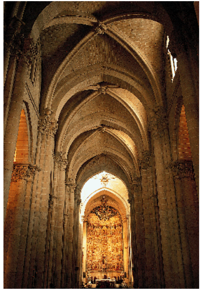
Interior de la nave mayor
