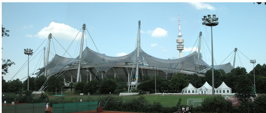
FIGURE 4. Otto Frei modeled the Olympic stadium in Munich on minimal surfaces. Image taken from http://www.archdaily.com/109136/ad-classics-munich-olympic-stadium-frei-otto-gunther-behnisch
